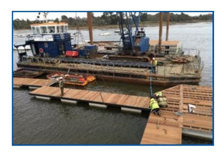
Our utilities contractor, Shoreline, will start on site this week and will commence all the wiring and plumbing whilst Walcon continue to weld the wall brackets back to the sheet piling at low water, the whole scheme is starting to look very smart and we are currently 10 days ahead of schedule.
